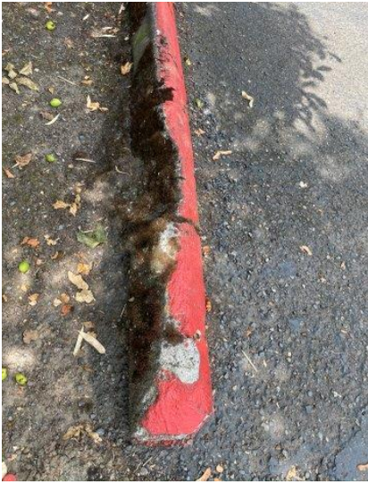
Concrete Safety Repair
