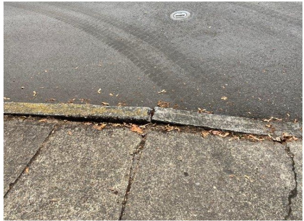
Concrete Safety Repair
